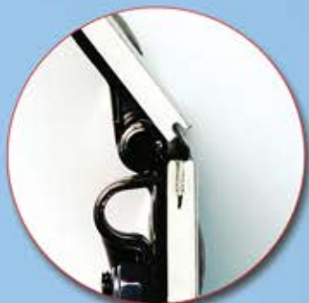
Tongue and groove panel with vinyl joint seal
